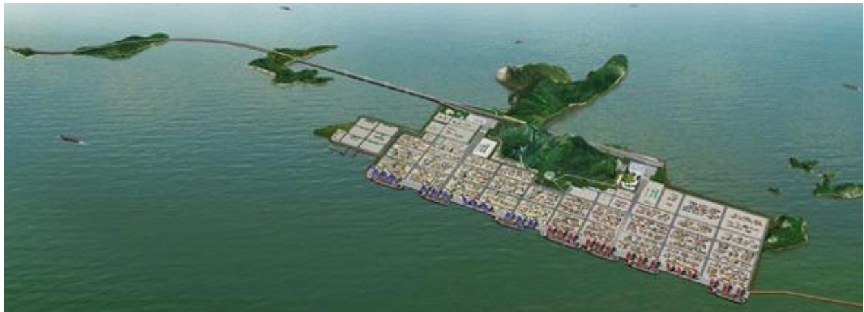
Figure 4. Shanghai Yangshan Deep Water Port
