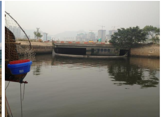
Stormwater Nullars (雨水渠)
